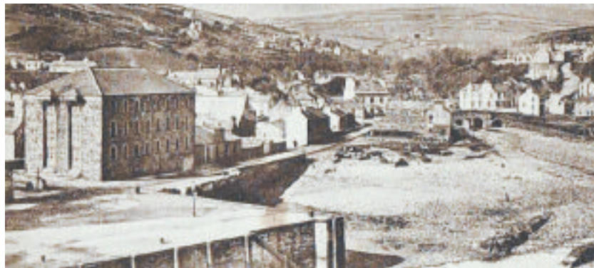
Laxey Pipe Factory, Williamson's behind
