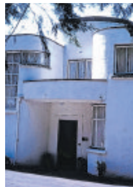
The front entrance to Ravenscourt. Note the curved glass in the windows and the central tower that lets light down into the circular hall below.
