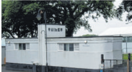
Designed by Leslie Hamilton Kearne A.R.I.B.A. the senior architectural assistant in the Borough Surveyor and Engineer's Department, this block stands close to the TT Grandstand. Note the period style writing on the upstand.
