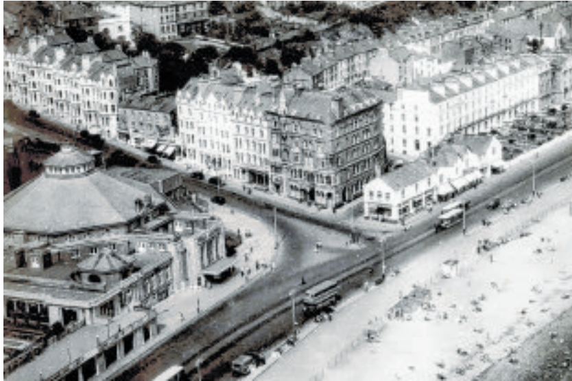
The end of Castle Mona Avenue with its entrance onto Broadway, prior to the demolition of the shops
