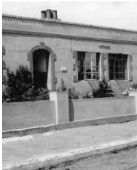
No 1 and 2 Hawthorn Villas on the Castletown Road as built by J C Barry and Sons. Many will recall them in the early 1970s as 'The Sizzler' restaurant before it moved to Onchan
