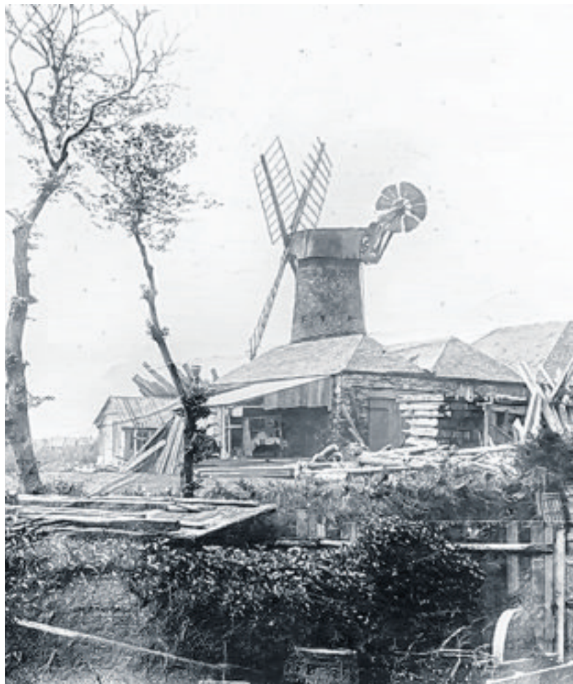
Kelly's sawmill in Kirk Michael with fantail, and inset the previous five-winged mill which burned down in 1865 (both iMuseum photographs)
