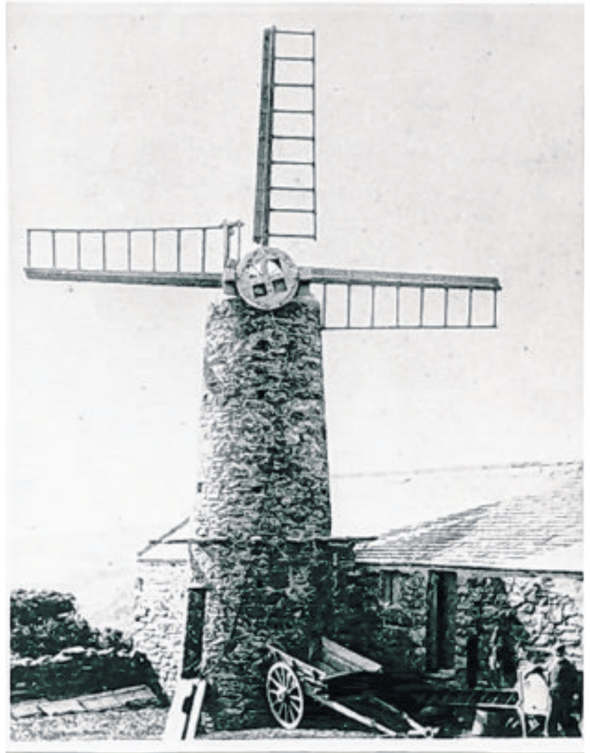
Baldromma, Maughold where the tower survives. The ring of projecting posts at barn-eaves level were used when rotating the head into-wind, and could also be used for support when the sails were rigged or reefed (Pic: iMuseum)
