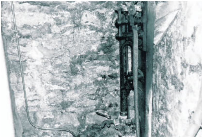
A hand-pump used to fill the track-side tanks; and the arrangements to transfer the contents to the engine. A long chain is pulled downwards which in turn lifts a big brass plunger in the bottom of the tank - like a bath plug - allowing the water out of the tank and into the locomotive (Picture: Sunnycroft collection)
