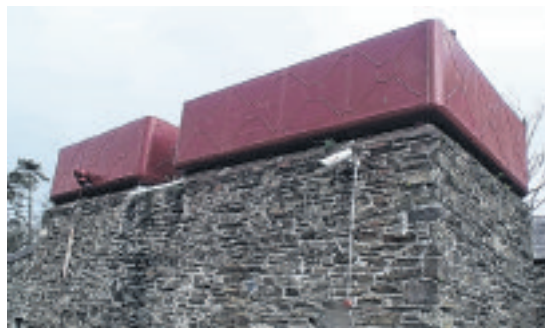
At Douglas station - Ransomes and Rapier water tanks filled by pumping river water until early 1980s
