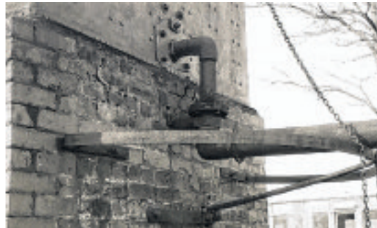
The riveted tank at Port Erin 1965 (Picture: John Maddrell)
