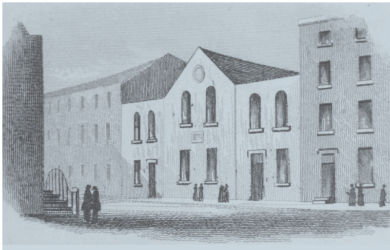
Independent Chapel, Athol Street, Douglas (demolished)
