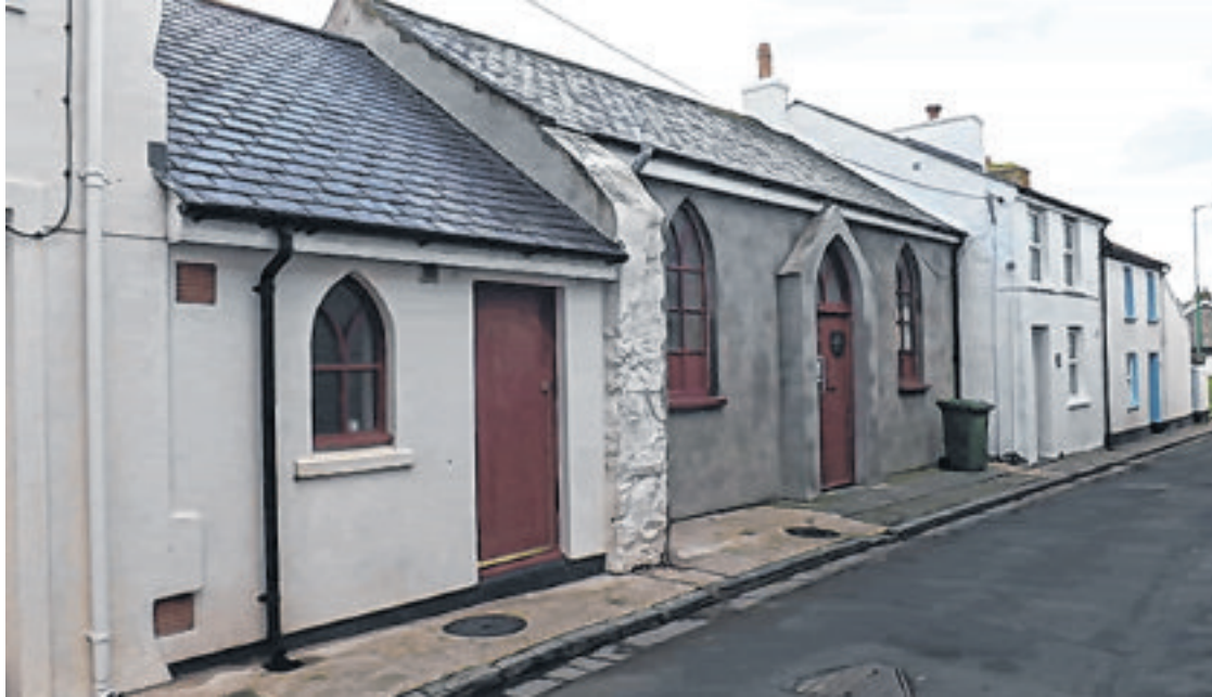
Queen Street Mission Hall at the heart of the street and the community, where the Roll of Honour was originally displayed - an example of a building that was at risk through loss of original purpose but has been saved, cherished and sympathetically extended by a community group who have given it a new life as the bandroom for the Castletown Metropolitan Silver Band (photo: Richard Hoare cc-by-sa/2.0)
