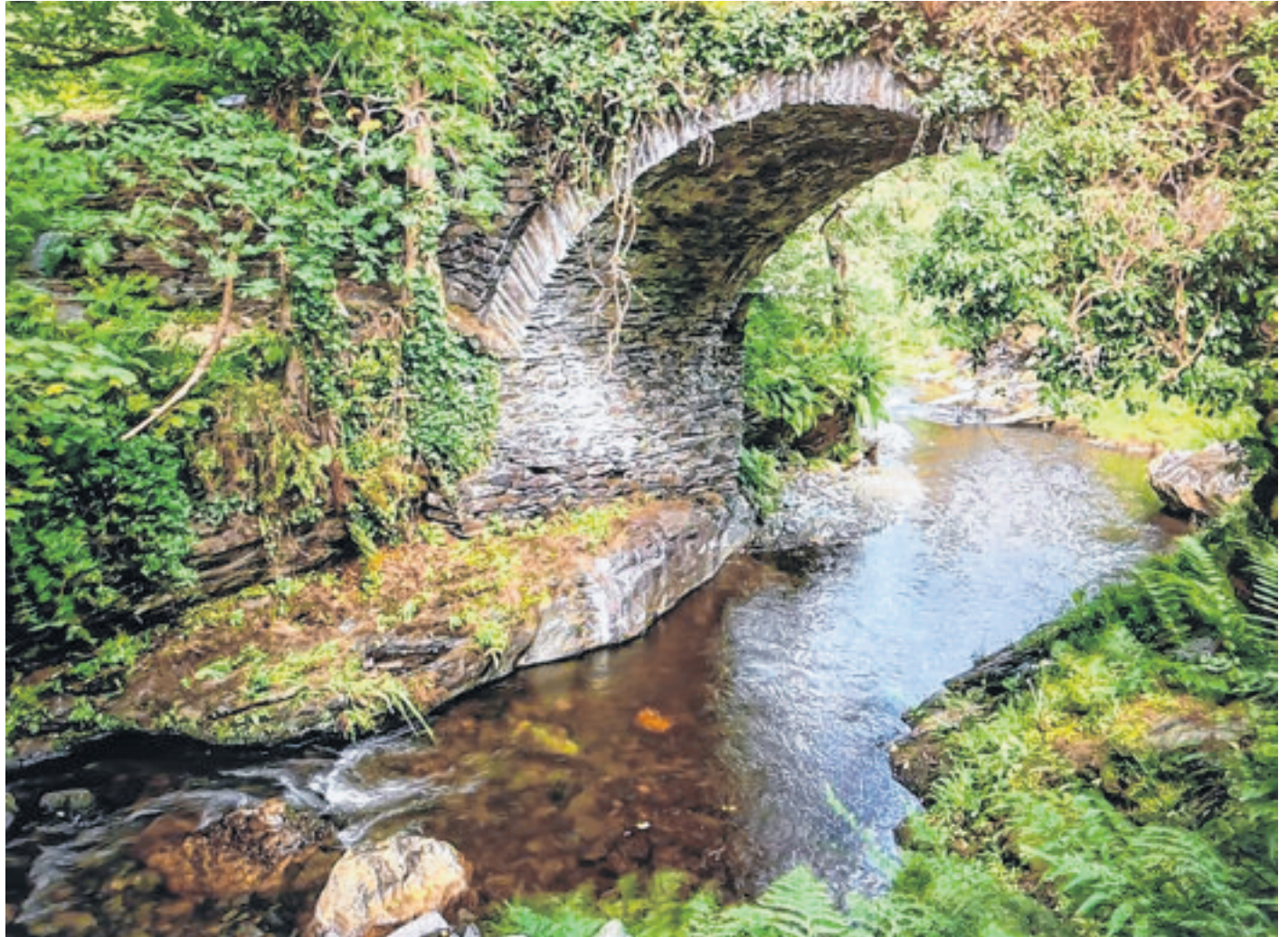
Ballakelle bridge (photo Don Smith)
