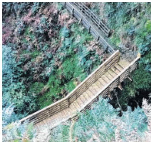
Tholt-y-Will glen: New bridge and its delivery via helicopter (DEFA)
