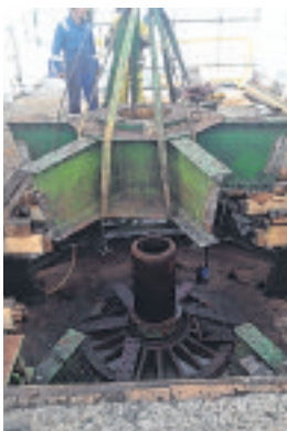
Repairs under way - dismantling the 120 year old bearing (photo: DOI)
