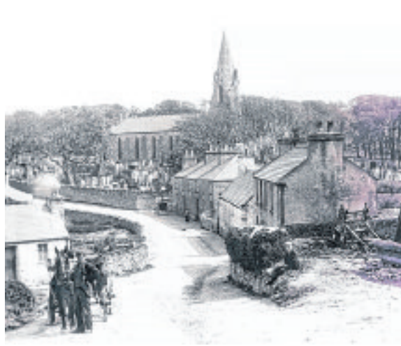
The Butt after the cottage was re-roofed in slate in 1900
