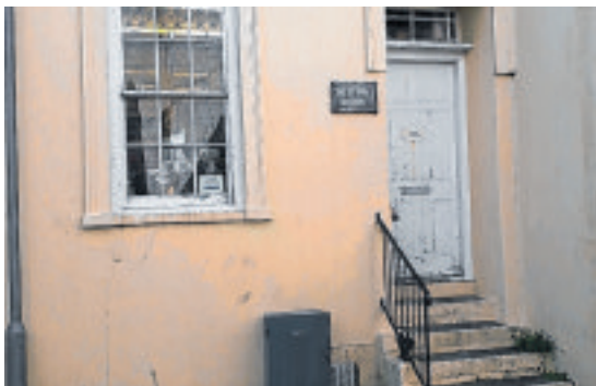
Castle Street entrance
