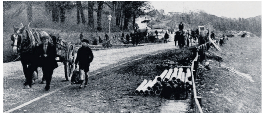
Widening Peel Road below Thornton in the 1930s. It was greatly widened on the south side between the 1830s and 1950s, but the stone retaining walls bounding the former mansion grounds follow the road's original course
