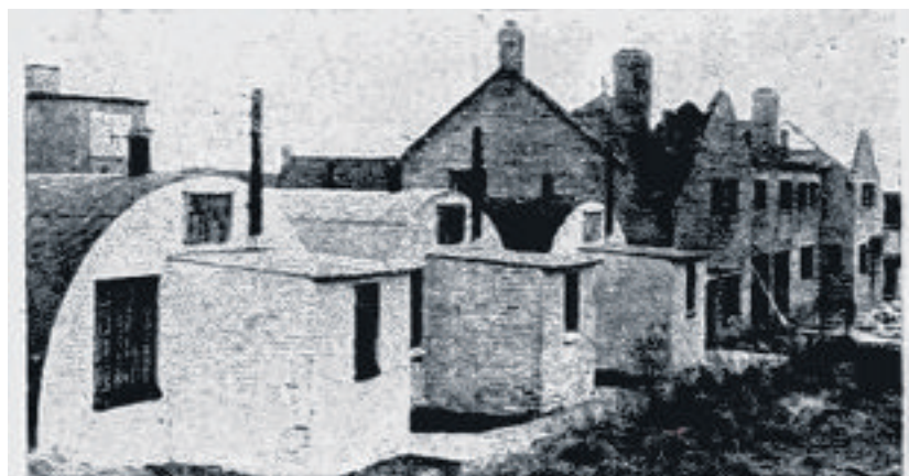
PROGRESS. — Nissen huts are giving way to permanent dwellings on the Ballasalla Temporary Housing Estate, and our picture shows how matters stand this week. The houses are being built to the order of the Local Government Board.
