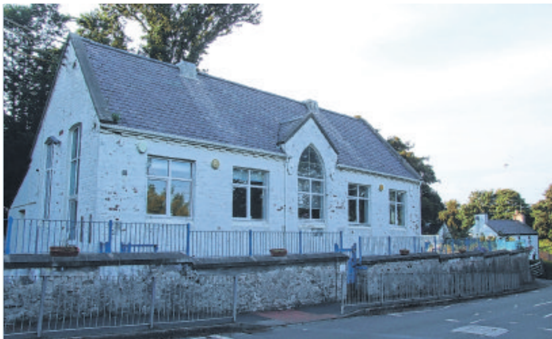
Bride School was built to accommodate the ever-increasing numbers of children in the parish but things have changed to the extent that Bride children now go to Andreas School. This was the only Parochial School in the north of the island built entirely out of local brick. Note the position of the former ventilators on the roof and how the original wooden window frames have been replaced with uPVC. Now the building lies empty
