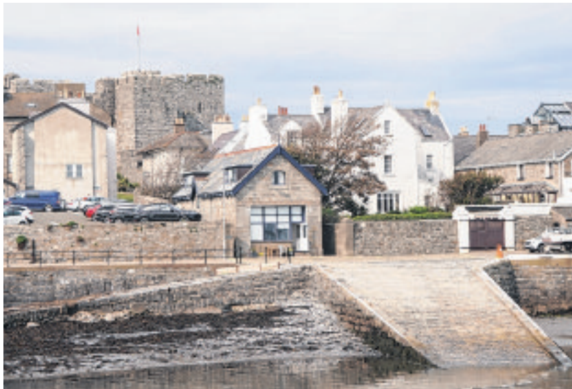
The second Castletown lifeboat house, now sympathetically converted to a dwelling
