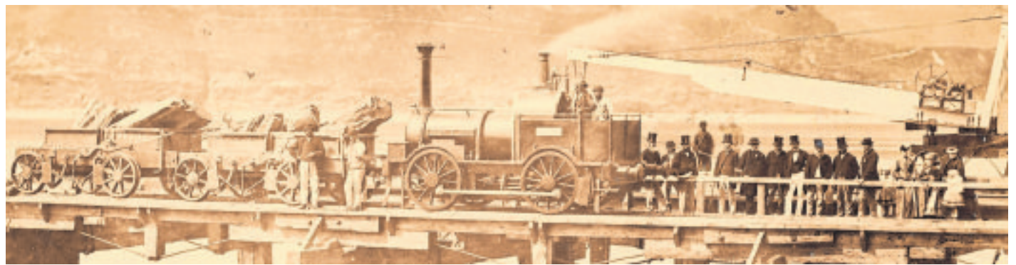
Building Port Erin's breakwater in 1864, broad-gauge engine and trucks with hand-operated tipping-beam crane behind (iMuseum)
