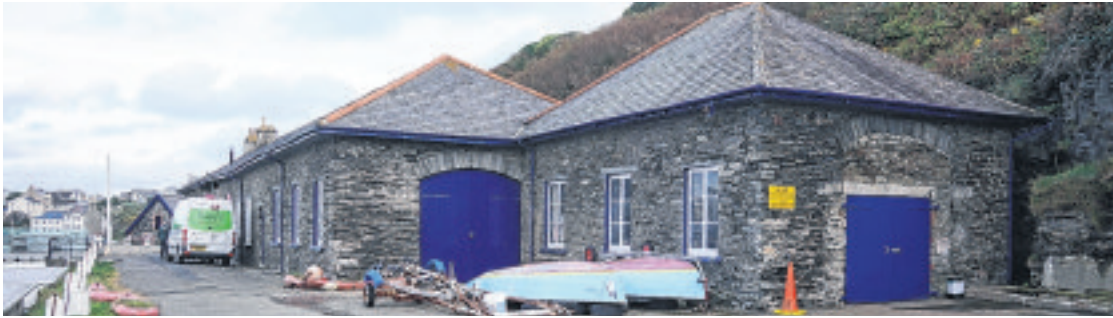
While the rails were lifted on completion and the engine shipped to Coođe's next project (possibly at Ponta Delgarda in the Azores), the Port Erin breakwater railway engine shed and workshop/blacksmiths survived and have various new sustainable lives
