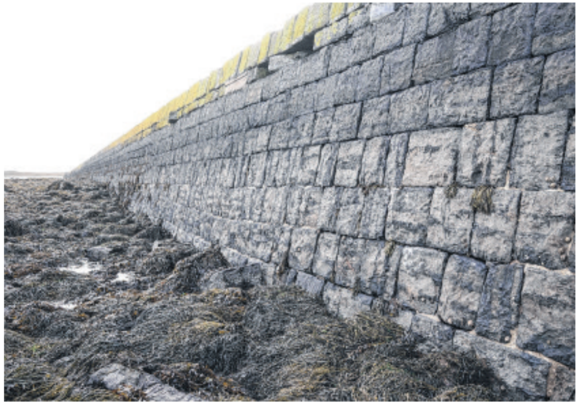
Derbyhaven breakwater – some sections still pointed, but others suffering from neglect and under threat of a 'concrete overcoat'
