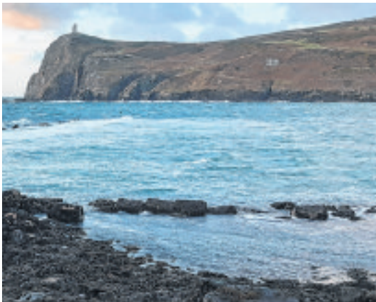
Even when partly wrecked, breakwaters can still have an effect. Waves rolling in from the southwest break and are reduced to just foam and spray inside the breakwater
