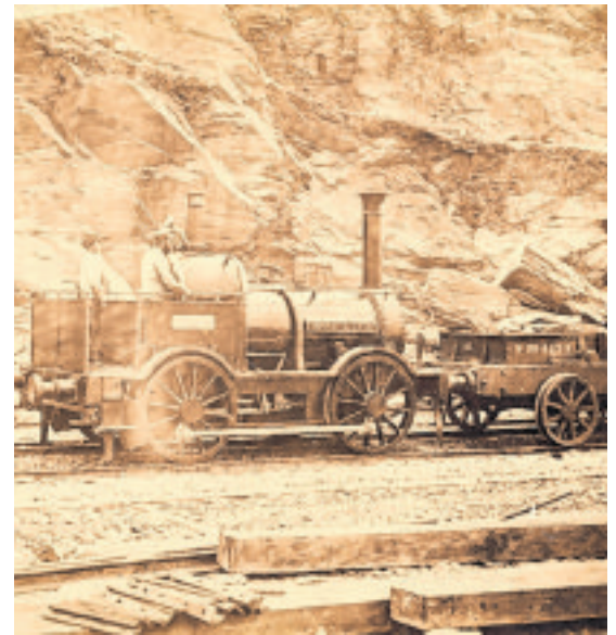
The massive rocks used to build Port Erin breakwater were hauled on the only Manx railway ever to use Brunel's Broad Gauge (7' 0¼") using an engine patriotically named Henry B Loch after the then Governor (iMuseum)
