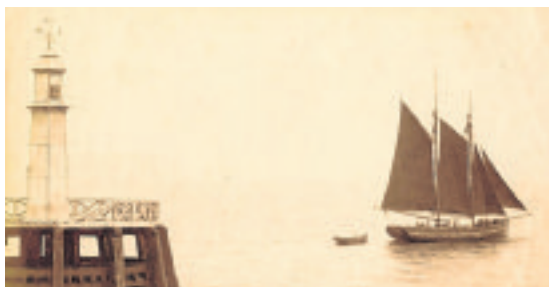
The first substantial light on Ramsey North Breakwater, atop the Abernethy birdcage breakwater structure. Those early light towers, assembled from a kit of iron panels, needed frequent attention to keep salt-water corrosion at bay (iMuseum)
