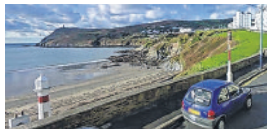
Port Erin leading lights – front light on the beach, rear light on the Promenade (Google Streetview)
