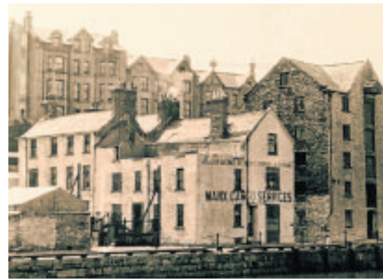
The former Holmes Brothers' house and Bank in the 1930s, described by the photographer John James Frowde as 'Holmes Bros Bank with the lid off' as demolition looks to have started iMuseum
