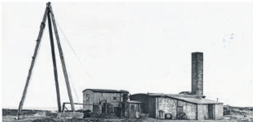
Pumping station in operation, looking east. The brine well is to the left underneath the sheer-legs used to raise the pump when it needed maintenance. The long connecting rod can be seen emerging from the engine shed and running to the inverted T-rocker at the head of the well - that inverted T-rocker converted the engine's horizontal stroke into the vertical stroke needed for the brine lift pump. The fresh-water pump can be seen at the extreme right of the picture
