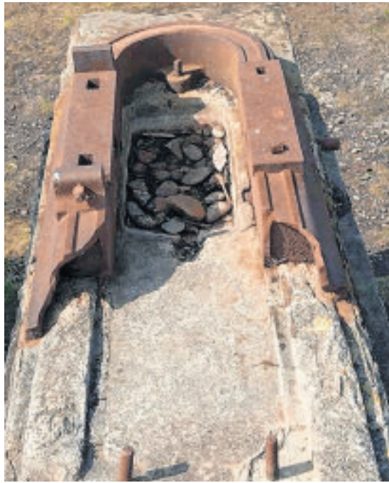
(Left photograph) the remains of the main lift pump engine bed and (right image) the connecting rod. (Inset) Pearn's double-ram banjo type combined engine pump, the type used to pump the brine from the settling tanks to Ramsey
