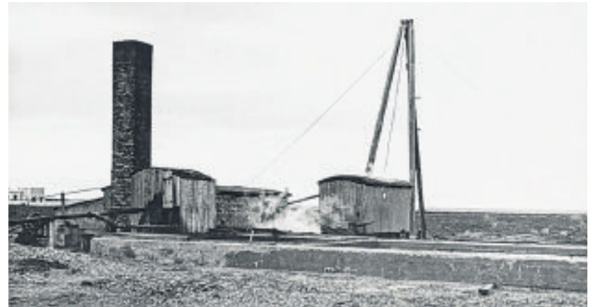
Pumping station in operation, looking west (lighthouse buildings visible far left of picture). In this photograph, the settling tanks can be seen in the foreground, with brine from the lift pump flowing into them, while the pipes from the delivery pump can be seen exiting the left of the picture at the start of the Ramsey pipeline
