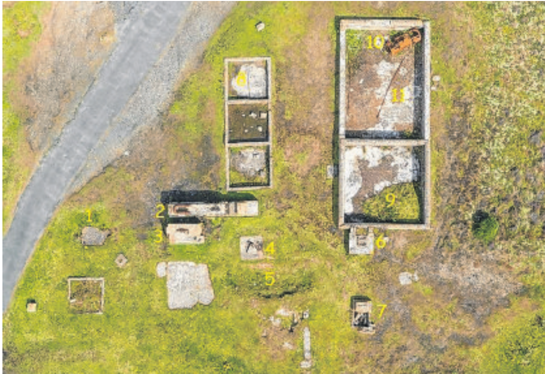
An aerial shot of the Saltworks which features the following: 1, deep bore brine well; 2, Well pumping engine bed; 3, Drive bed for pump rod; 4, Support column for steam pipe; 5, Boiler bed; 6, Brine output pump; 7, Fresh water well and pump; 8, Settling tanks; 9, Brine holding tanks; 10, Header tank for boiler feed; 11, Connecting rod between engine and well head
