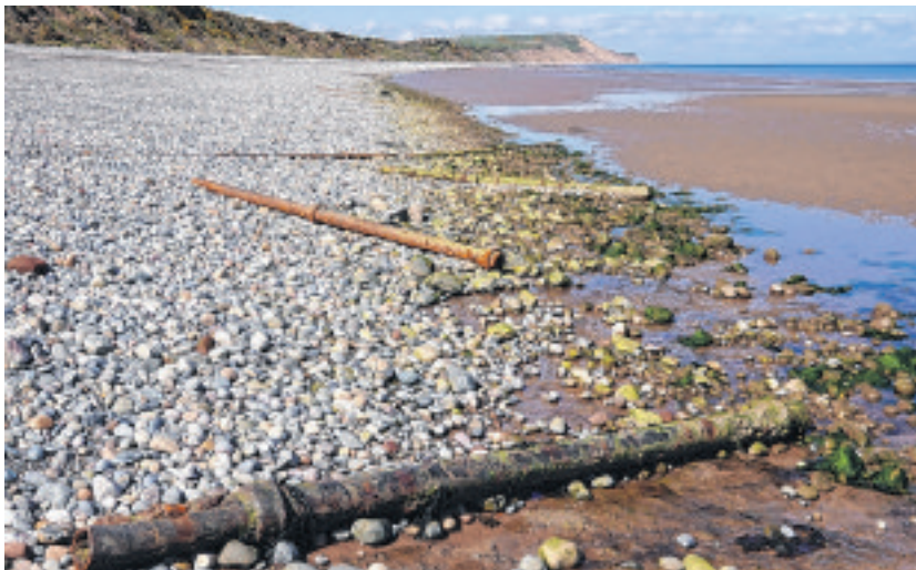
Segments of the pipeline strewn across the beach by wave action
