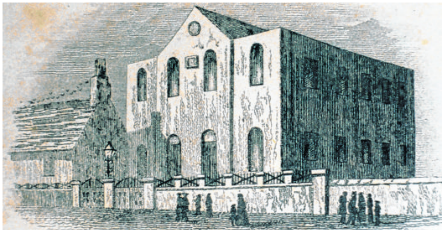
The original Douglas Methodist chapel is seen to the left of its replacement
