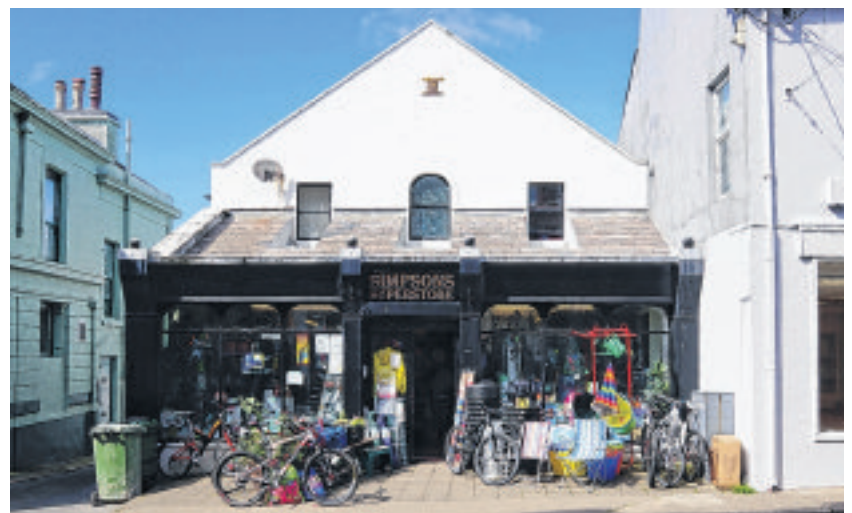
New life – the former Primitive Methodist Chapel in Michael Street, Peel
