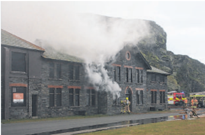
Marine Biological Station – not registered, neglected and now threatened with inappropriate and over-tall redevelopment
