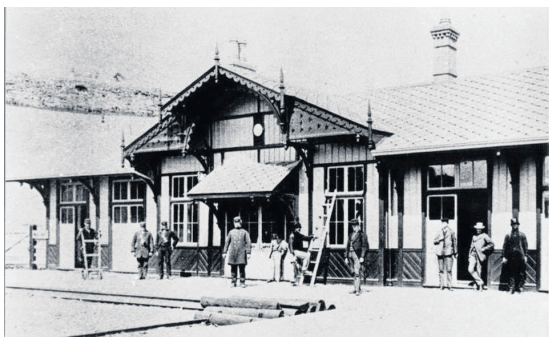
A close-up view of the first Douglas station, with its overhanging eaves and decorative front gable. End gables had filigree style decoration
