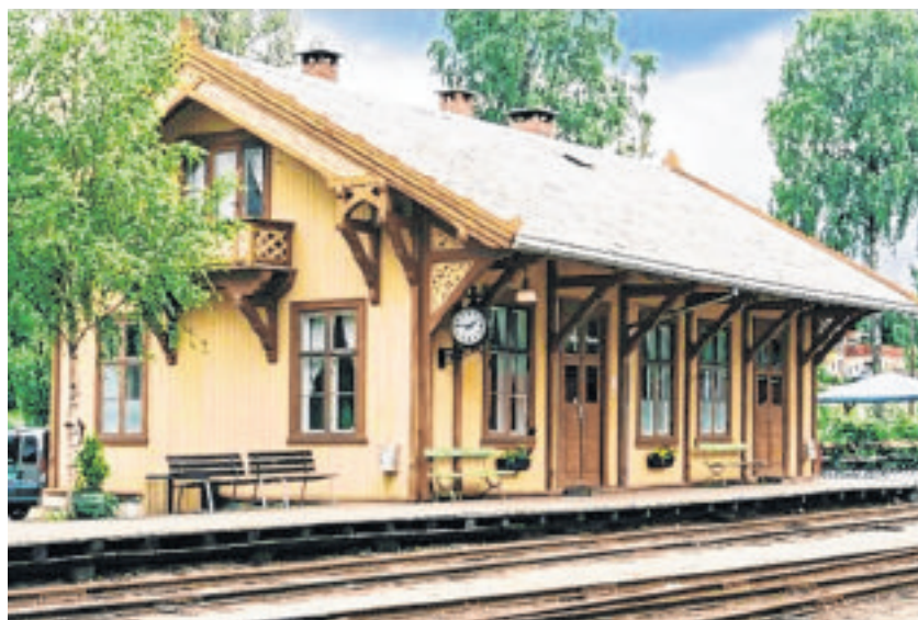
The surviving Kroderen station building in Norway has a similar look to the old Douglas buildings
