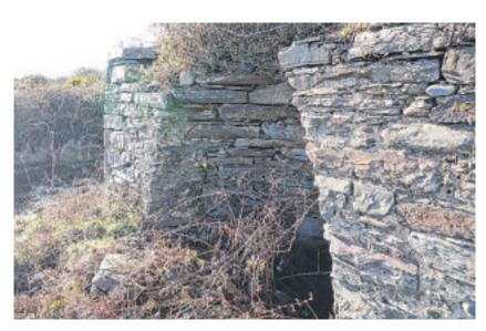
An early limekiln on the Ayres below Ballagarrett, Bride – note that the stonework has only been bonded with clay, although it has later had a coat of lime render
